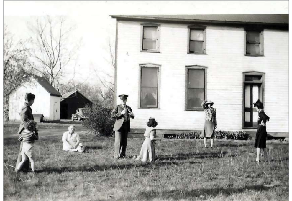
View of the cabin in 1945 with the family gathering around in front to welcome Cy Kinsella home on leave from the war. The cabin was rebuilt in 1976 shortly after the City took over to help extend the life of the last remaining structure on the farm. Eventually in 2023, the originally 160+ year-old wood logs had finally deteriorated enough that the cabin needed to be demolished for the safety of the public.
