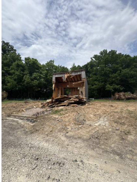
Demolition of the playground restroom in progress.
