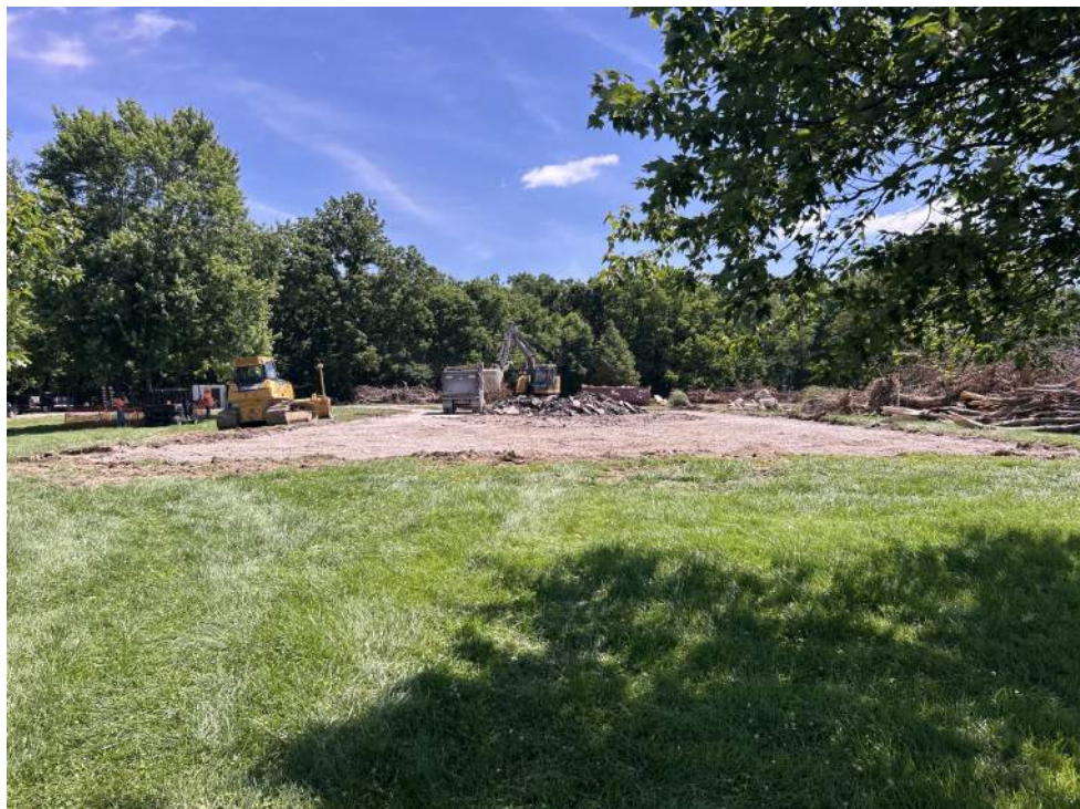
Asphalt removal at the park pavilion.
