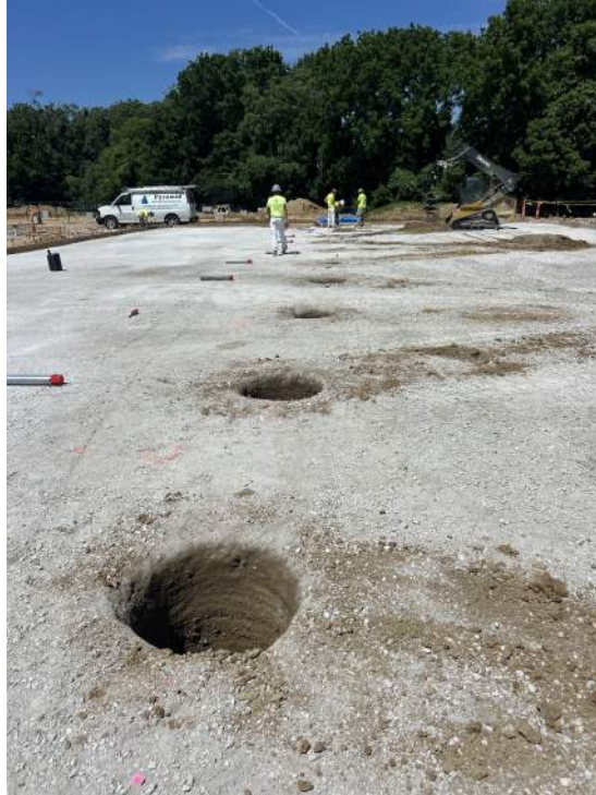
The interior post-tensioned slab during sleeve boring.
