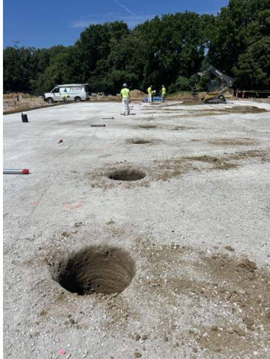
The interior post-tensioned slab during sleeve boring.
