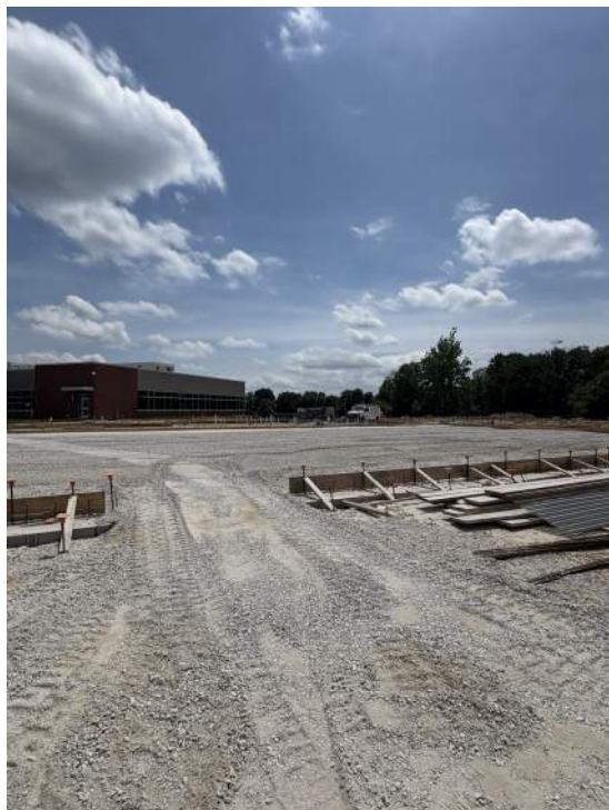
A view of the Rec post-tensioned slab after rock grading.
