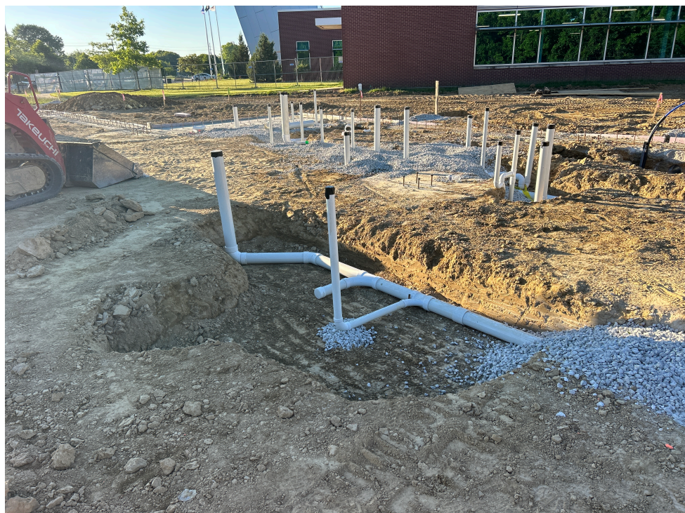
A view of plumbing underslab rough-in at the main building prior to slab placement.
