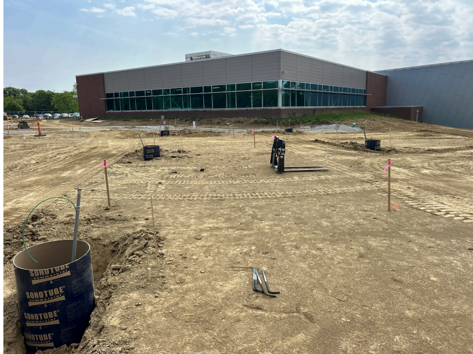
Light pole bases set at the outdoor court.
