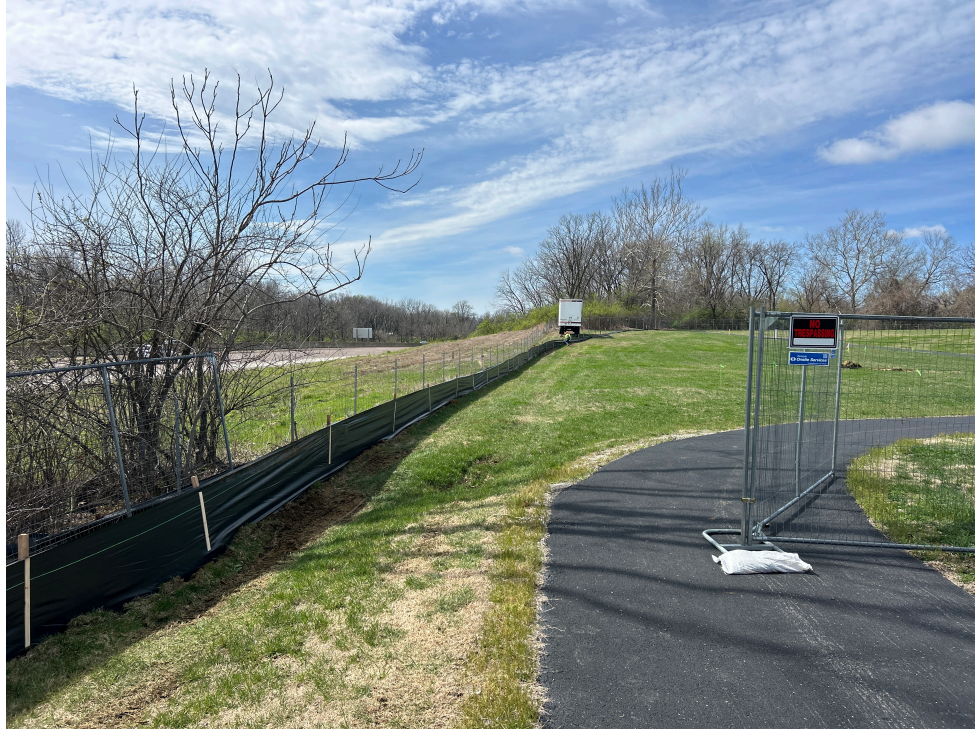
A view of the newly installed silt fence.
