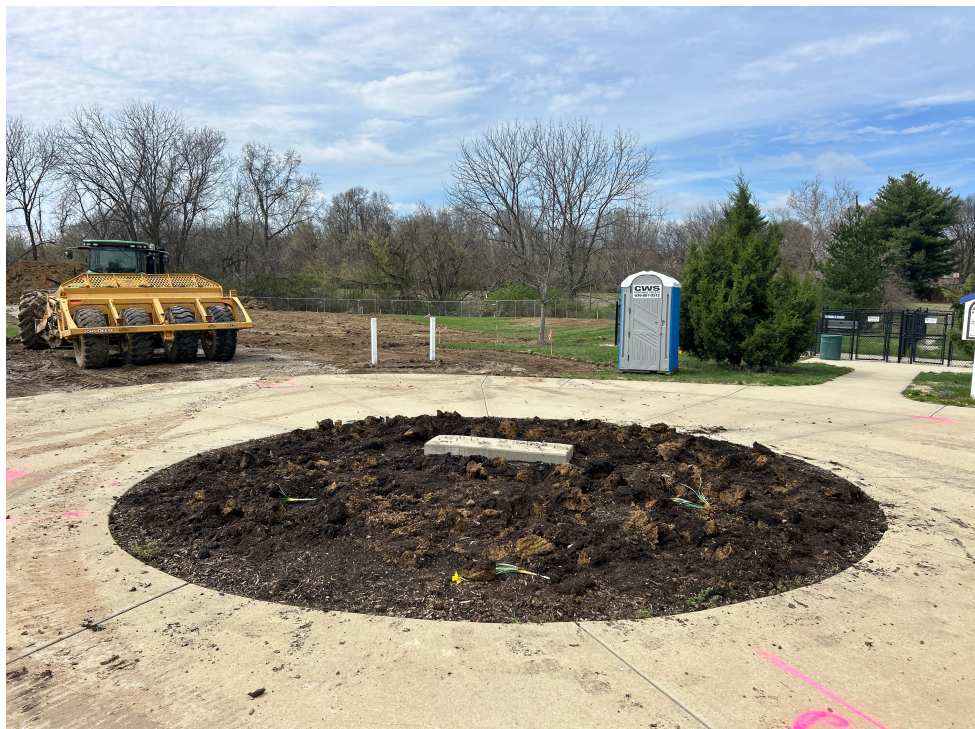
The sidewalk after demolition began and the sign was removed.
