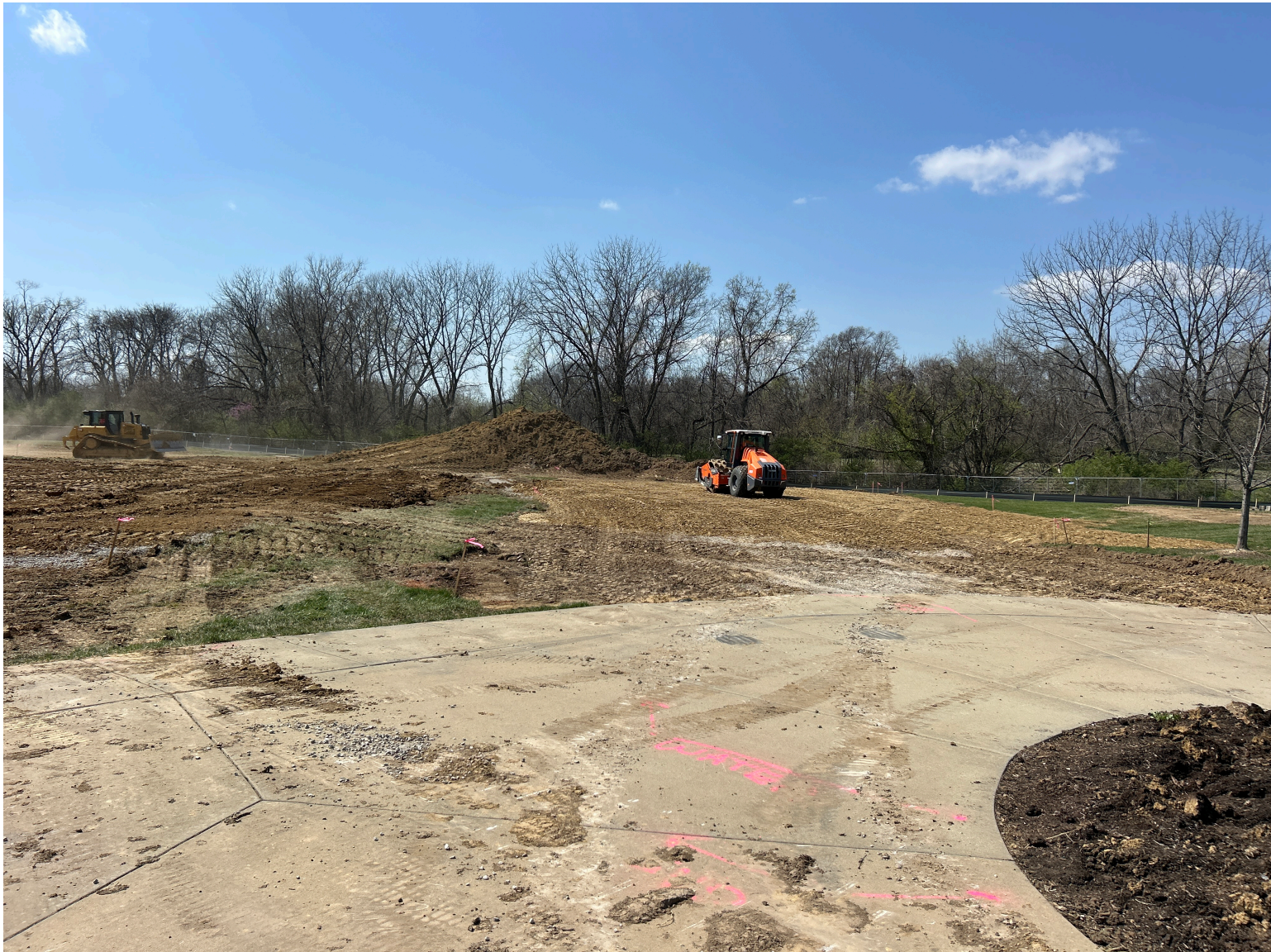
A photo of ongoing compaction for the new parking lot and continued site grading.
