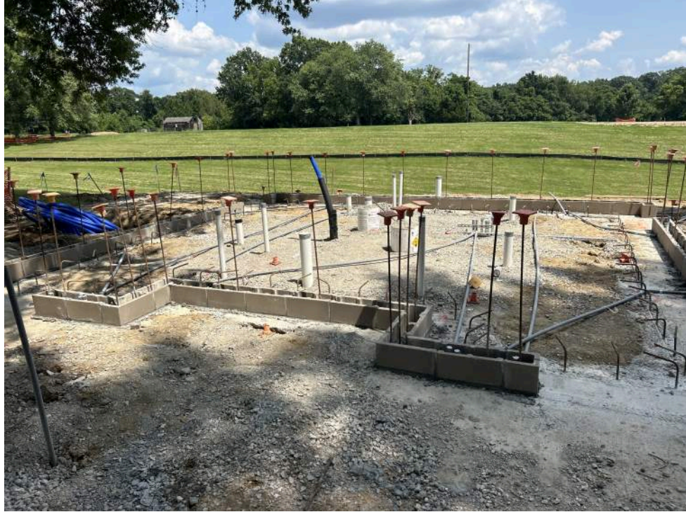
A view of the first course of block and underslab electric at the special event restroom.
