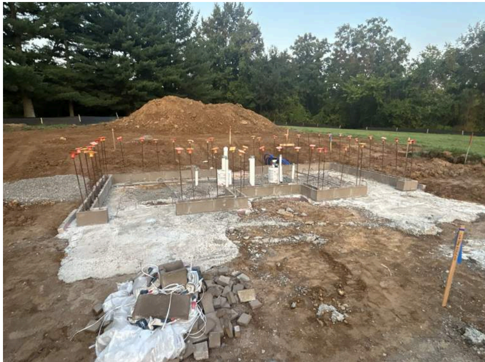
A view of the first course of block and underslab electric at the Dog Run.
